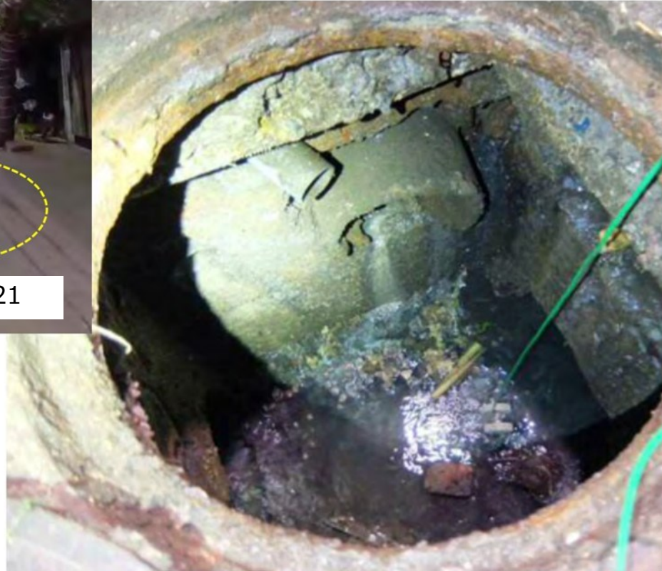
Corroded manholes before replacement
