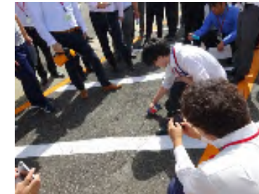
ひび割れ補修剤注入を実演
