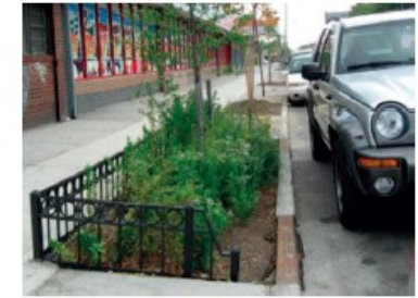
Commercial Corridor: Post-Construction Enhanced Tree Pit
