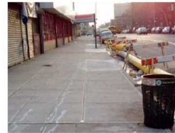
Commercial Corridor: Pre-Construction
