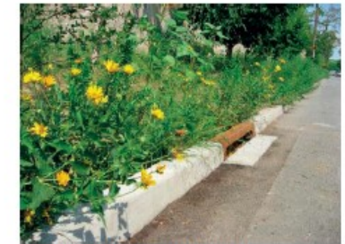
Low Density Residential Street: Post-Construction Infiltration Swale
