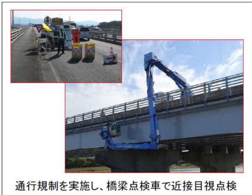
従来点検 (H26～H30: 1巡目点検)
