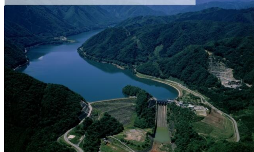
An aerial photograph showing a large concrete dam structure across a river valley. The reservoir behind the dam is a deep blue color, surrounded by steep, forested mountains. The surrounding landscape is rugged and green.
