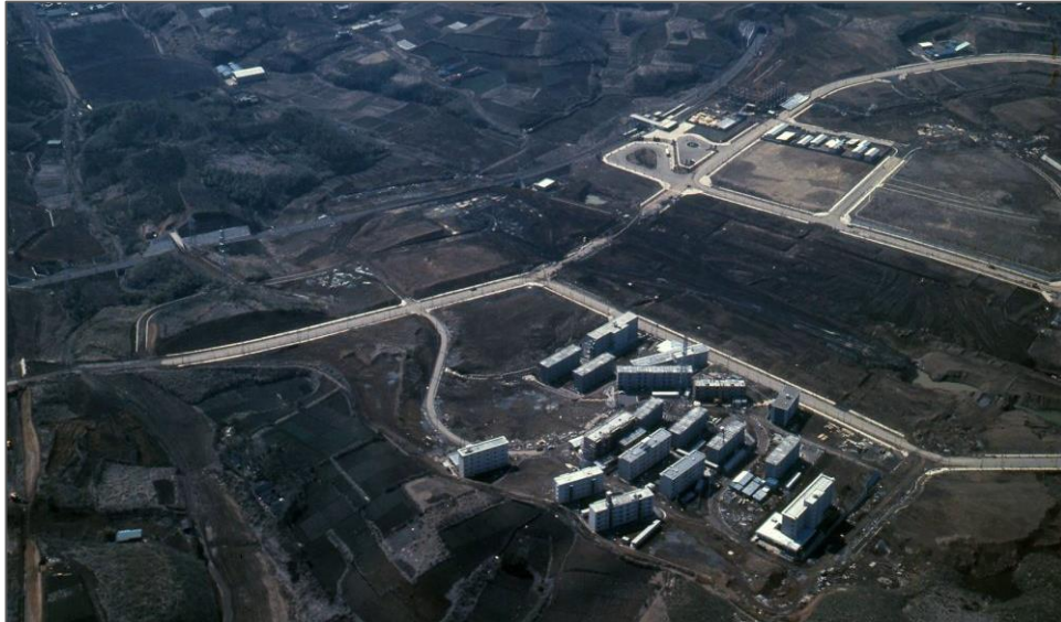
Site in an early phase of development (Tama-Plaza Station vicinities)
