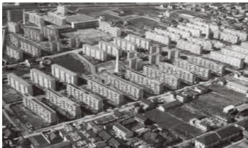
First JHC rental housing built in 1950s (Kanaoka Housing Complex, Osaka)
