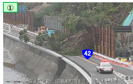
① 法面崩落の状況(R4.6) [串本町上浦地先]
