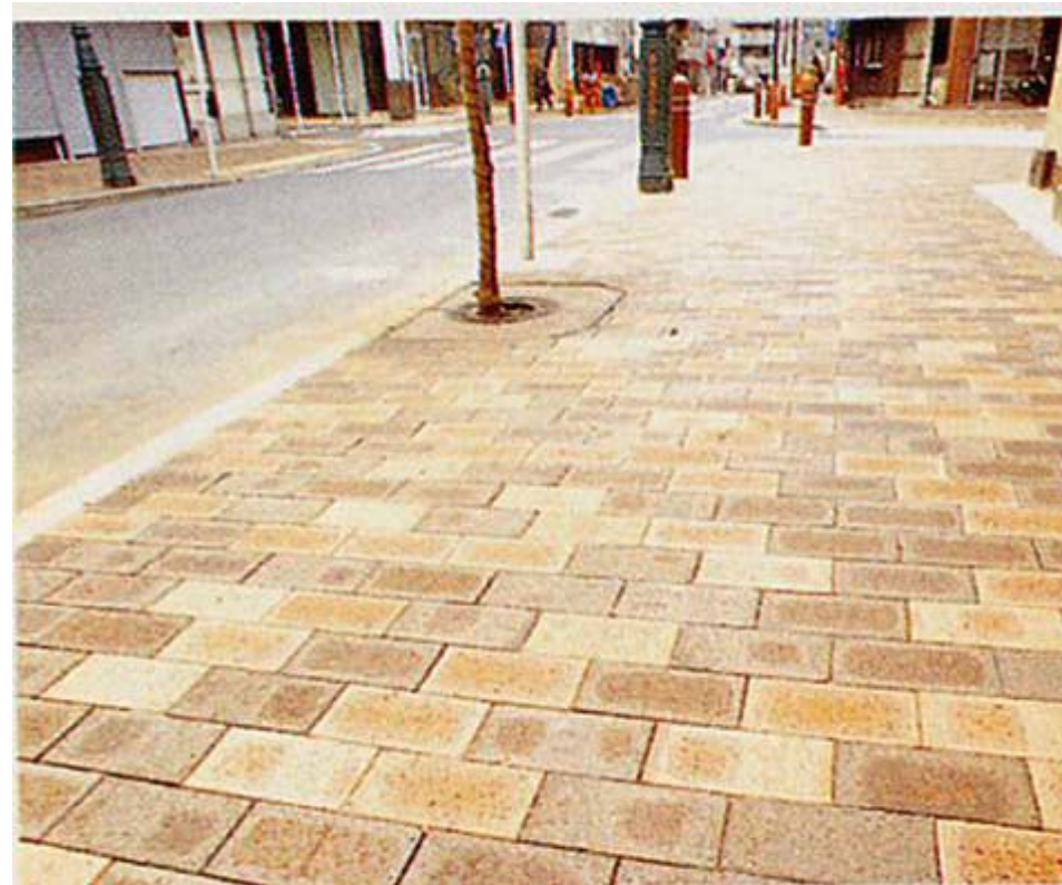
permeable tile pavement
