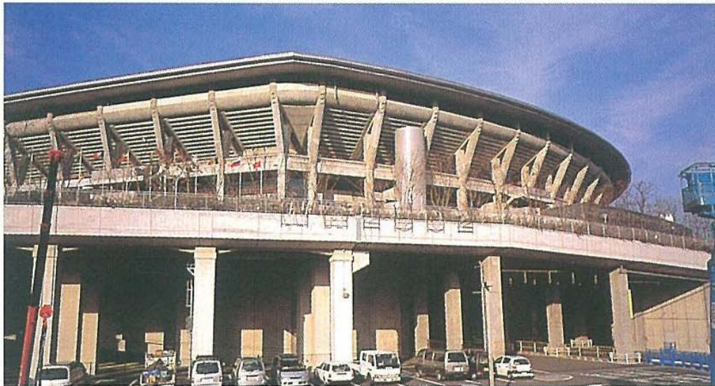
Pilotis structure employed for Nissan Stadium
