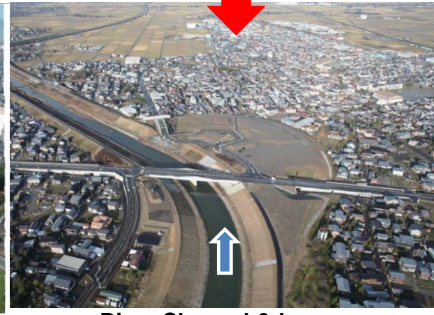
River Channel & Levee Improvement (December 2010) 44
