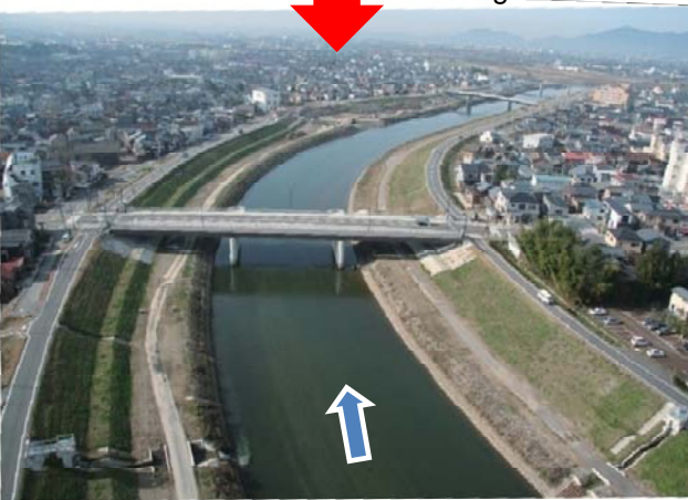
Widening & Excavation (December 2010)
