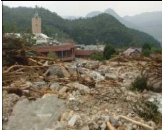
Damage of a special nursery home for the elderly
