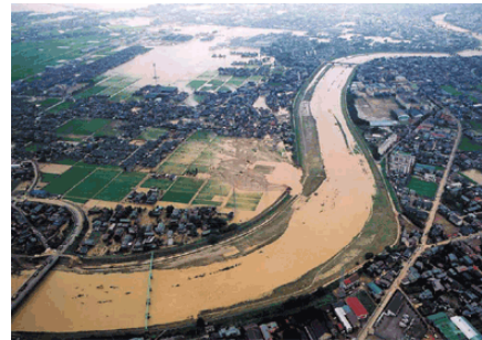
Overflowing of smaller rivers (Ikarashi River) (July 2004 Niigata-Fukushima Flood Disaster)
