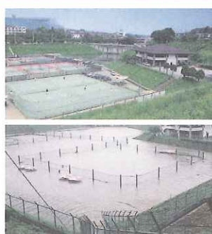
Tennis court with flood control function. Flood damage is mitigated by controlling runoff into river at storage and infiltration facilities (Ex. School, park etc.)
