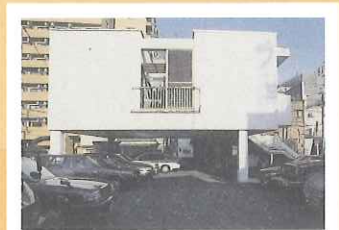
Piloti-type structure for flooded damage mitigation.
