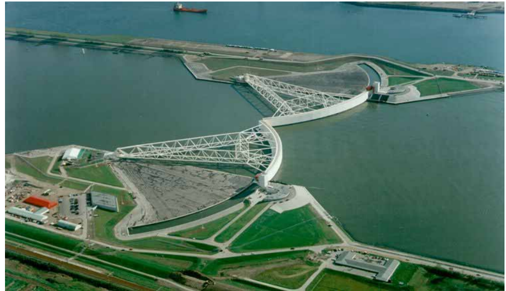
Maeslant Storm Surge Barrier)
