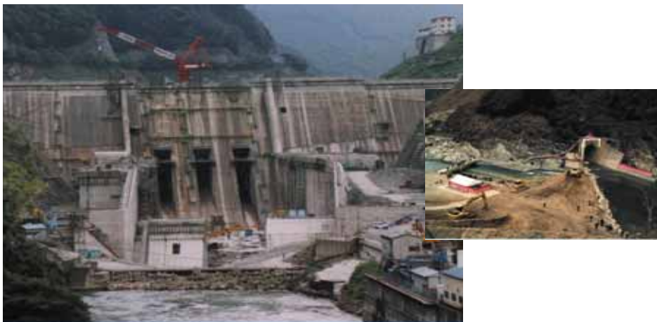
Construction of a flood-regulating dam
