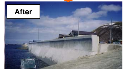
Rehabilitation of aging revetment by setting up anterior wall
