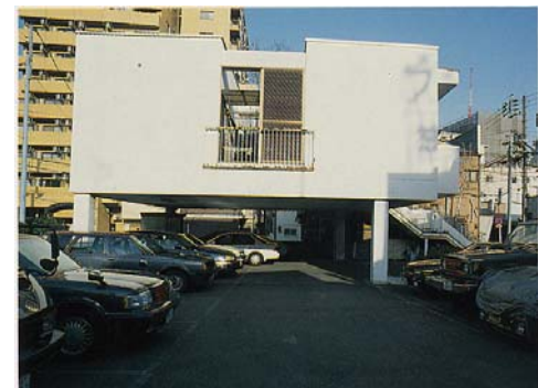
Adopting pilotis to prevent damage to buildings during a flood
