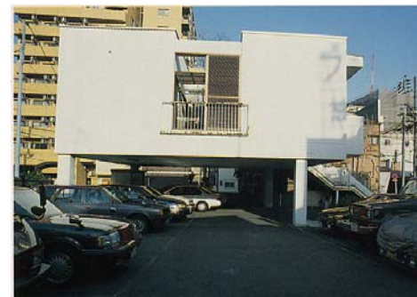
Piloti-type building to avoid damage during a flood
