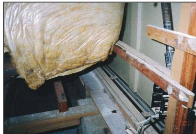
Having absorbed water, insulation materials have become useless.
