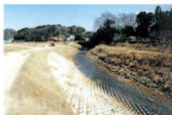
(Below) Before work Shallow and flat flow. Connected blocks exposed on the slope
