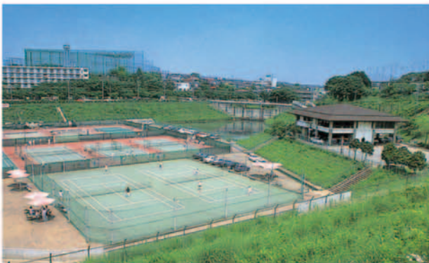
Kirigaike regulating reservoir, Kanagawa Prefecture This is normally used as a tennis court.
