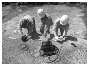
護岸の点検・補修
