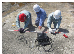
護岸の点検・補修
