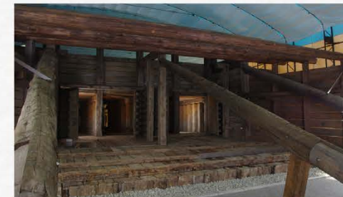
Restored exhibit of the Kanamawari Shiken Monpi sluice gate
