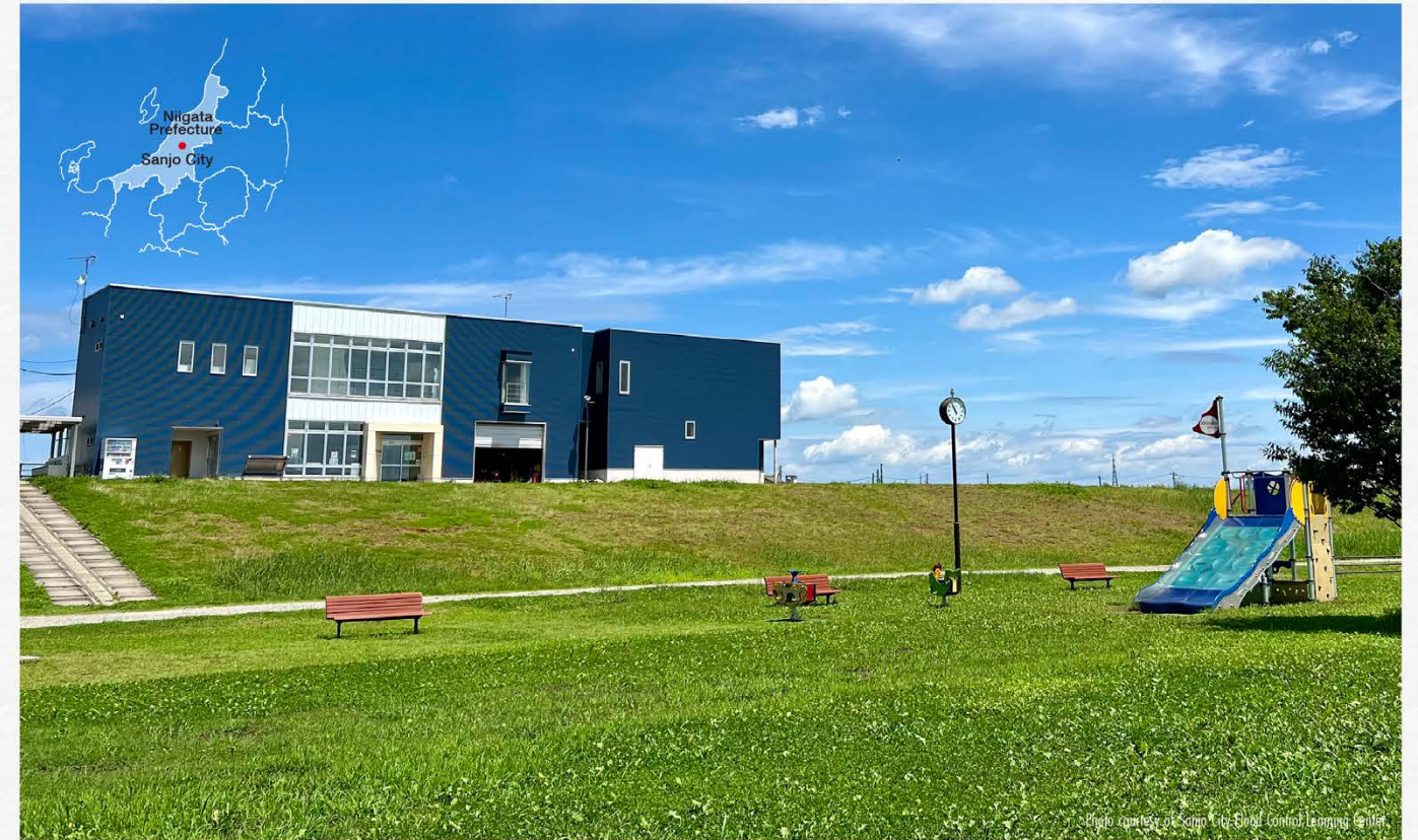
Photo courtesy of Sanjo City Flood Control Learning Center
