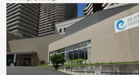
Exterior of the Tsunami/ Storm Surge Disaster Prevention Station
