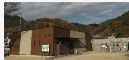
Exterior of Saka Town Disaster Densho Hall located inside the park
