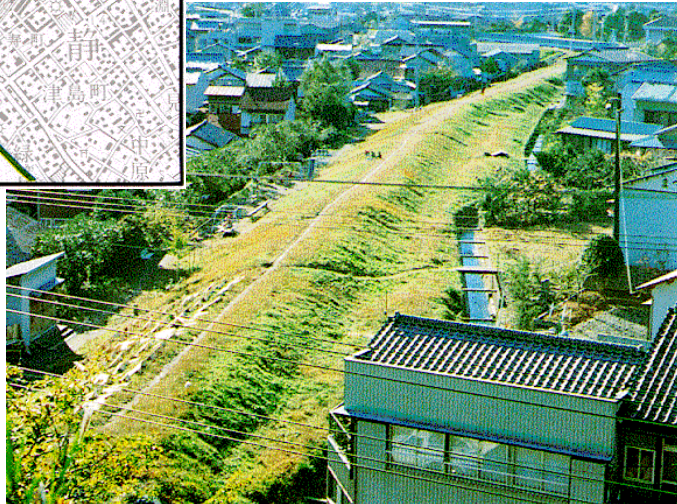
The surviving part of the Satsuma Levee(bank)
