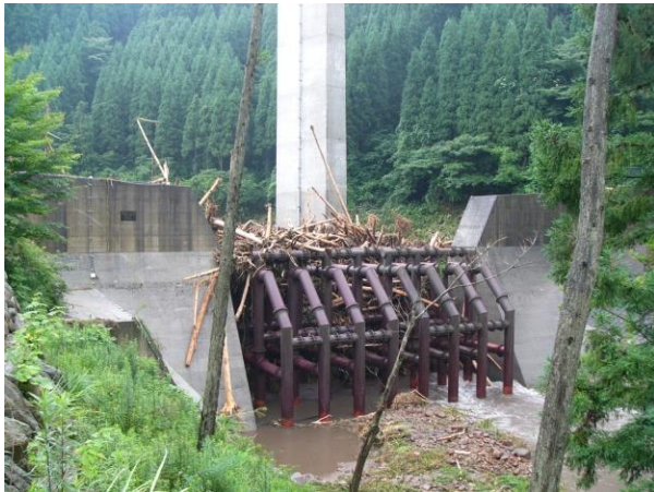
<Installation of check dam to capture debris flow>
