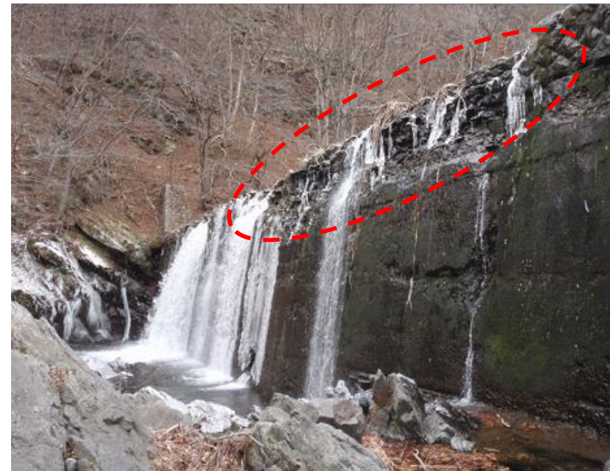
Erosion of the crown of check dam,
