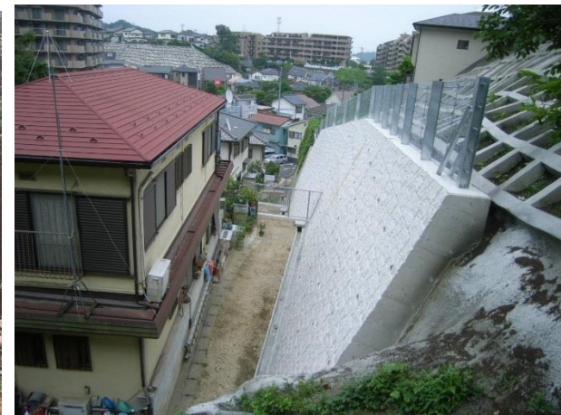
<Installation of retaining wall to prevent slope failure>
