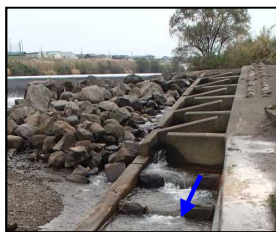
左岸魚道改修前 (H26)
