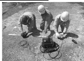
護岸の点検・補修
