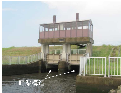
樋門樋管の事例(利根川太田排水樋管)
