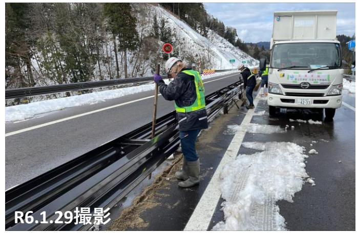
No.14 段差補修状況
