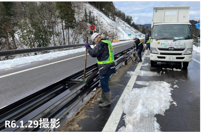
No.14 段差補修状況
