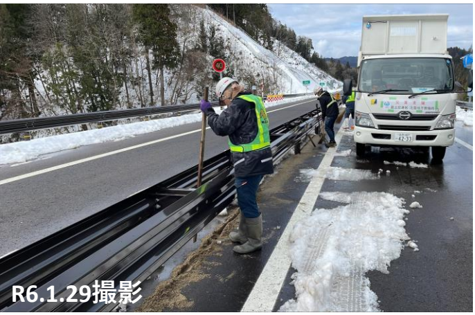
No.14 段差補修状況
