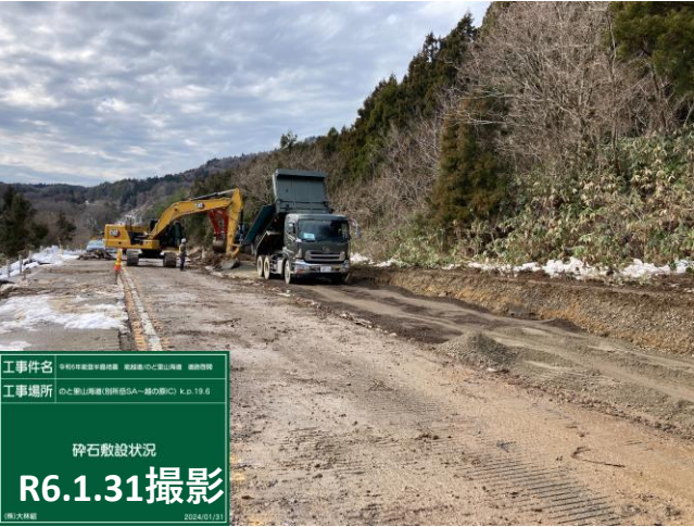
No.16碎石敷設状況
