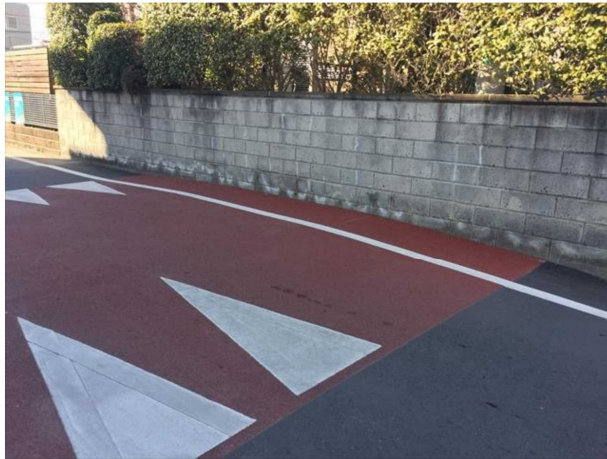
側溝上も併せて嵩上げ
