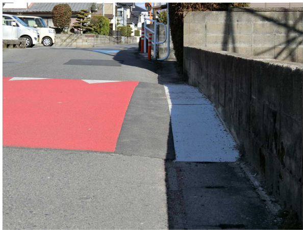
側溝上も併せて嵩上げ
