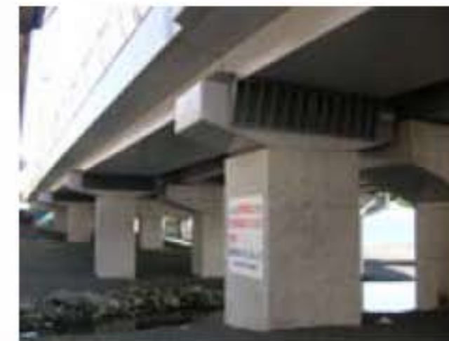
Jacketed columns and connecting superstructures
