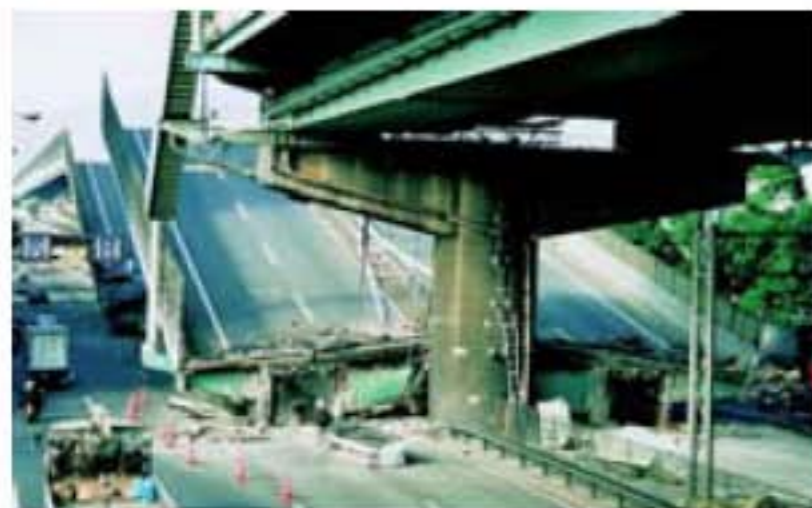
Damages by Hanshin-Awaji Earthquake (1995)
