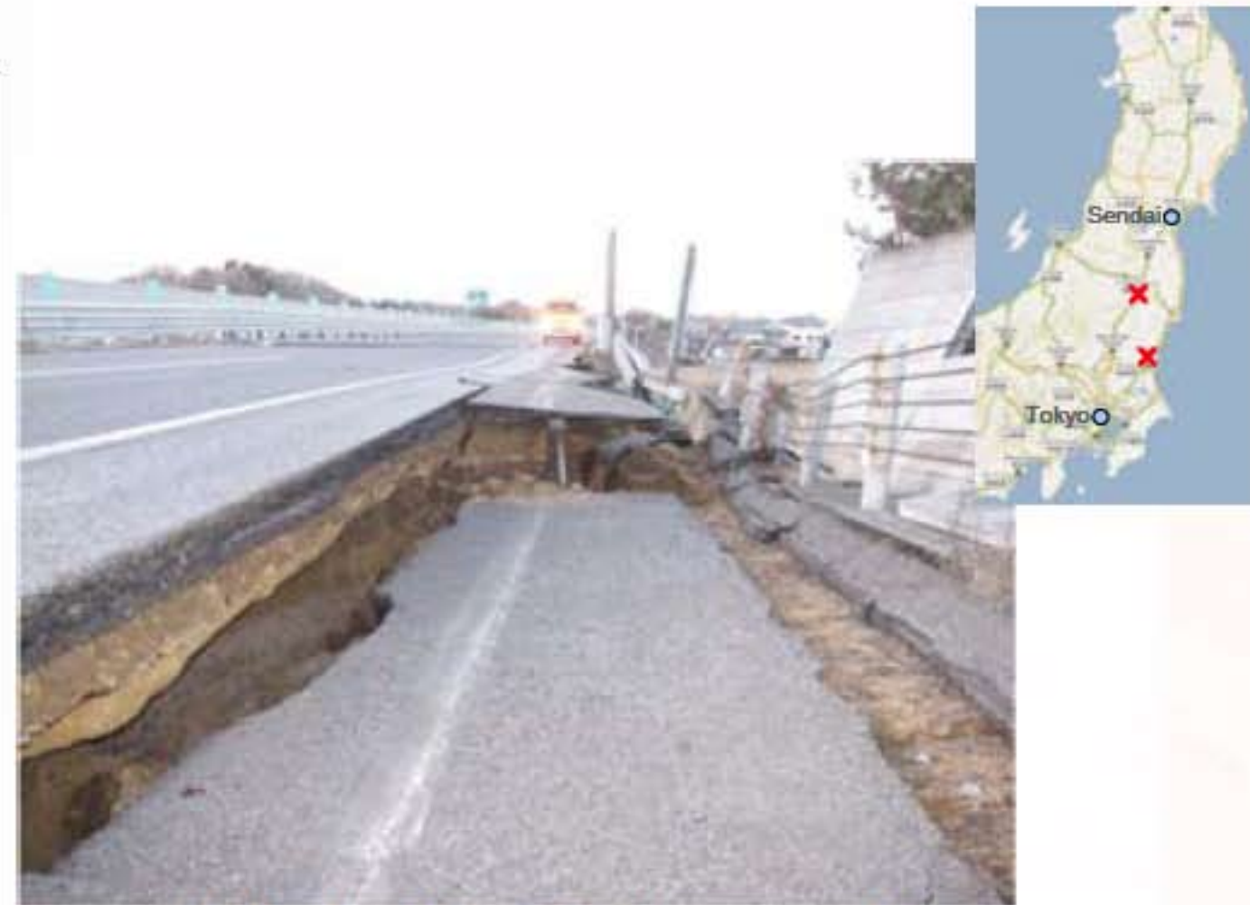
Yabuki IC – Sukagawa IC (Tohoku expressway)
