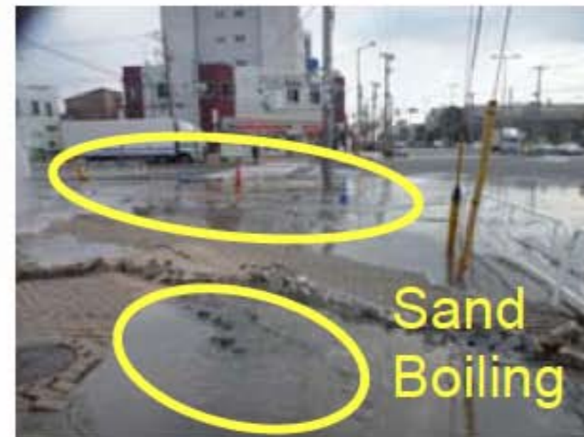
Sand boiling in reclaimed land
