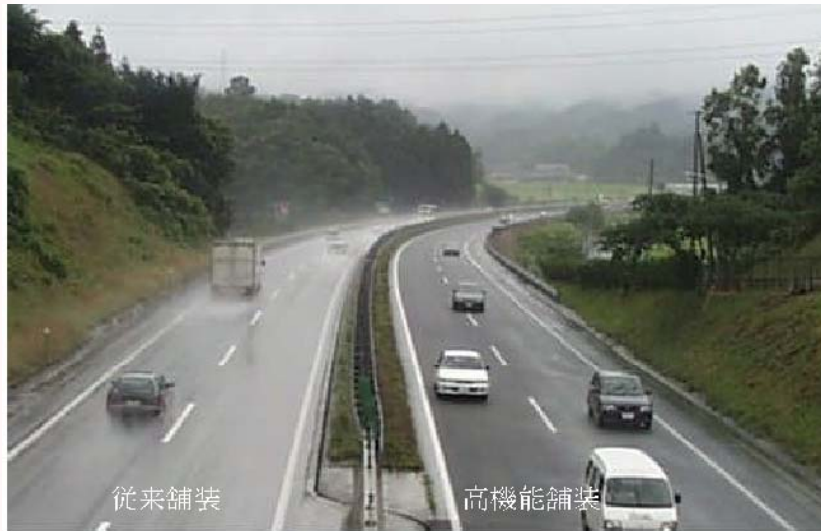
Old type pavement High Performance Pavement
