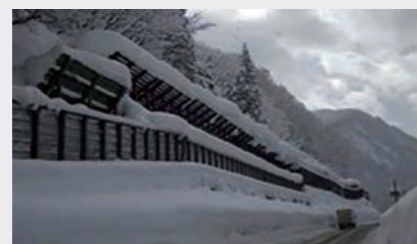
Snow protection work (Hokuriku Regional Development Bureau)
