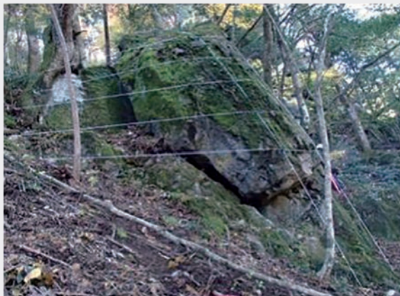
Wire rope work
