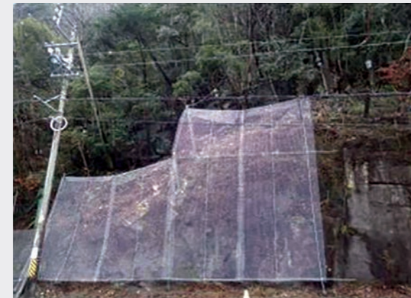
Pocket-type rock falling protection net
