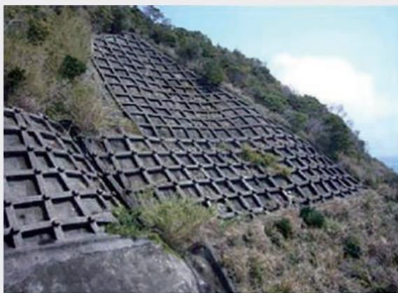
Crib work + anchoring
