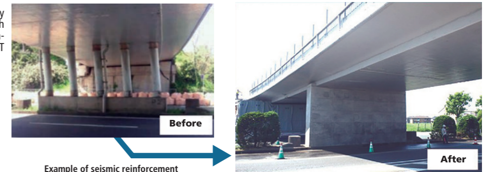
Example of seismic reinforcement
