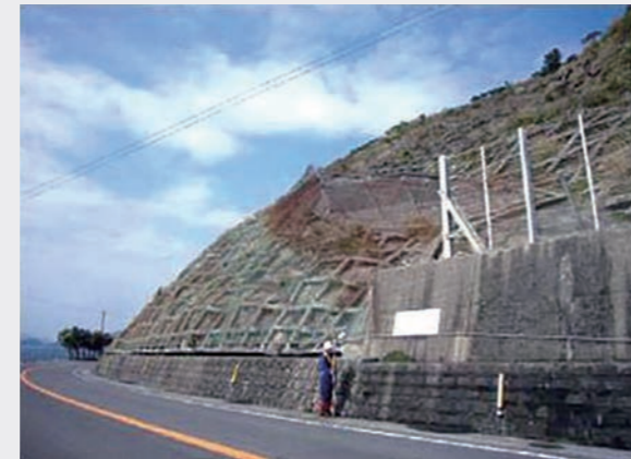
Concrete crib work
