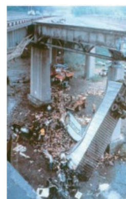
Collapse of the Maianas Bridge (1983)
