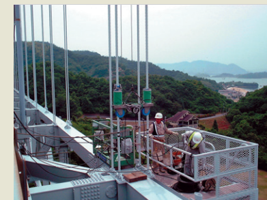
Non-destructive inspection of hangers
