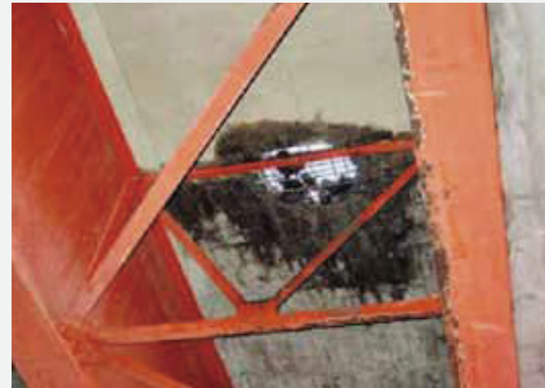
Collapsed slab due to fatigue
