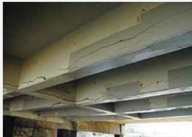
Deterioration due to salt damage
