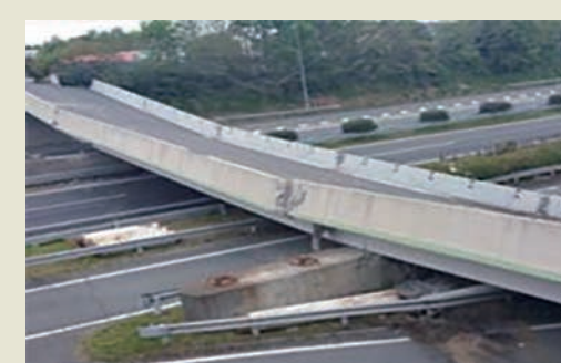
(1) Collapsed a rocking pier over Kyusyu Expressway (Prefectural road Ogawa-Kashima Line, Furo Daiichi Bridge)
