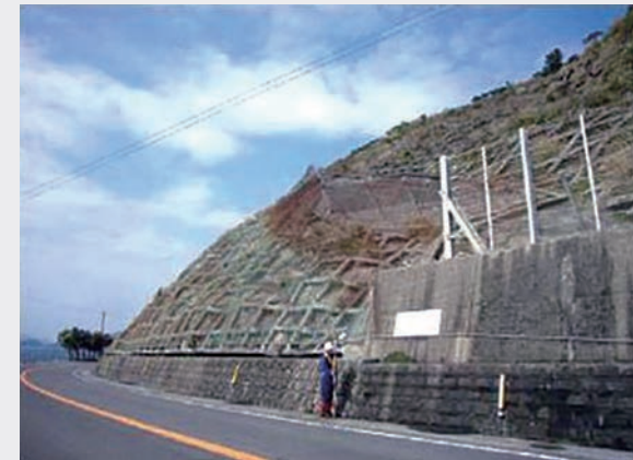
Concrete crib work
