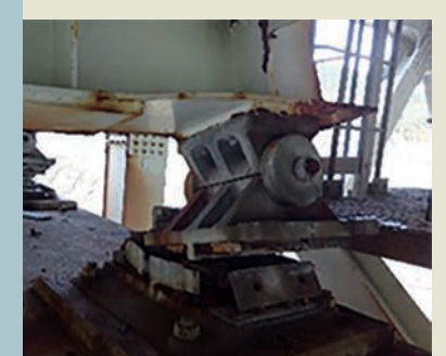
(3) Damages on supports and main girders of a bridge (Heiryu Bridge, Oita Expressway)
