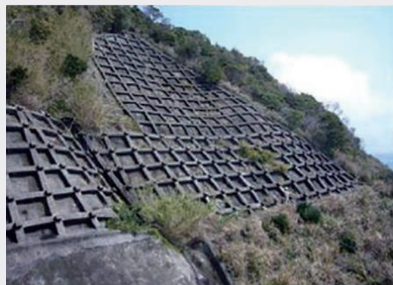
Crib work + anchoring
