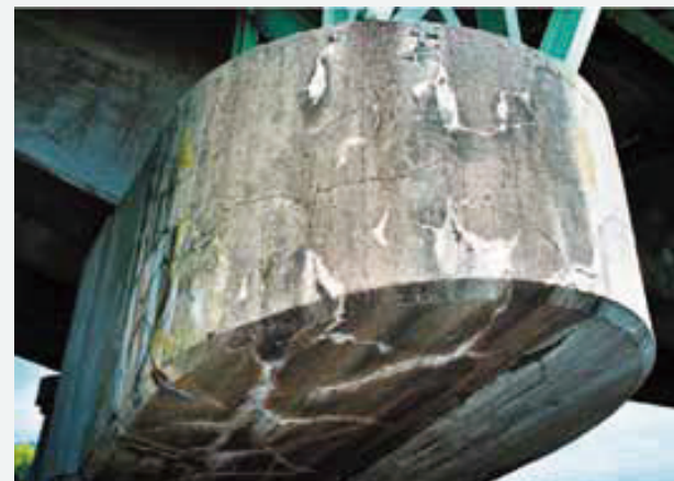
Deterioration due to an alkali aggregate reaction
