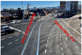
Verification of support measures at complex intersections (image) (Maintenance of demarcation lines to be detected by in-vehicle sensors)
