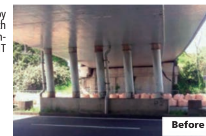
Example of seismic reinforcement
