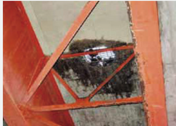
Collapsed slab due to fatigue
