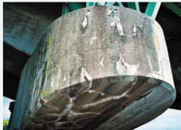
Deterioration due to an alkali aggregate reaction
