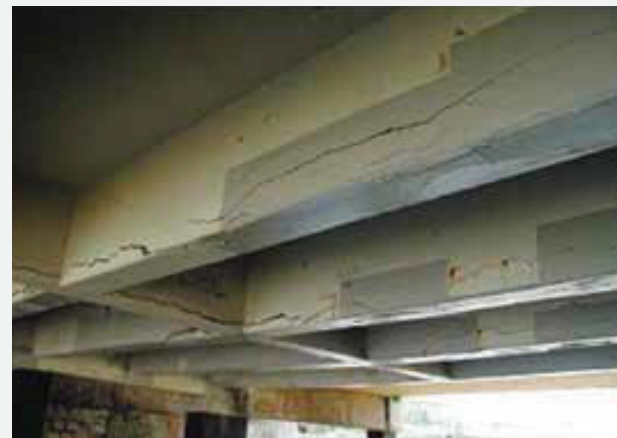
Deterioration due to salt damage
