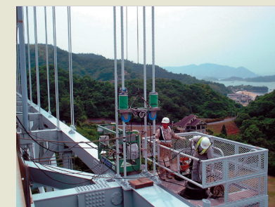
Non-destructive inspection of hangers
