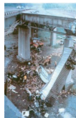
Collapse of the Maianas Bridge (1983)
