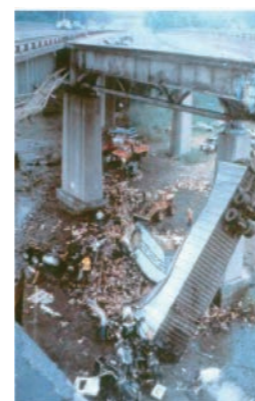
Collapse of the Maianas Bridge (1983)
