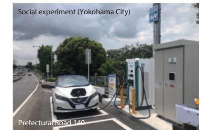
Installation of EV charging facilities on public roads
