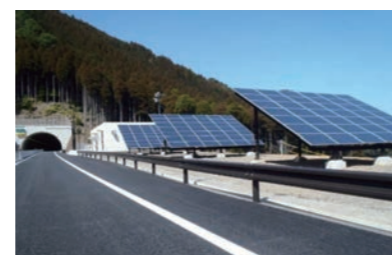
Solar power generation in road space
