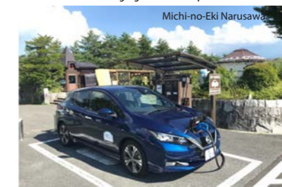
Installation of EV charging facilities at Michi-no-Eki
