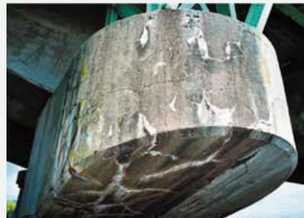
Deterioration due to an alkali aggregate reaction
