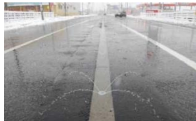
Provision of snow-melting facilities
