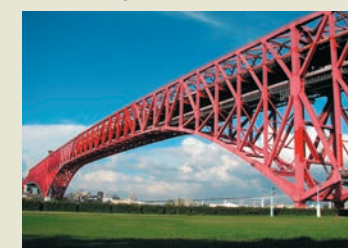
Use of a damage control earthquake-resistant design on the Minato-ohashi Bridge helped reduce the construction cost (Hanshin Expressway).
