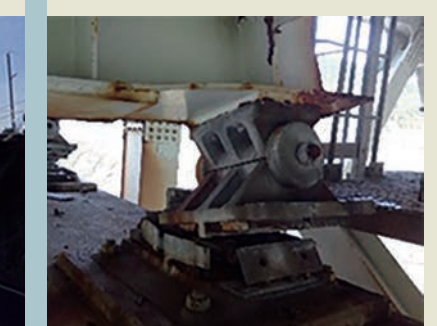
(3) Damages on supports and main girders of a bridge (Heiryu Bridge, Oita Expressway)
