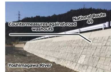
Countermeasures against road washouts on National Route 49 (Iwaki City, Fukushima Prefecture)
