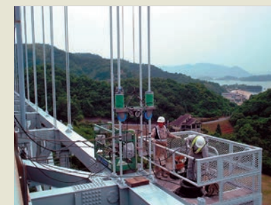
Non-destructive inspection of hangers
