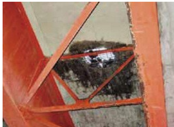
Collapsed slab due to fatigue
