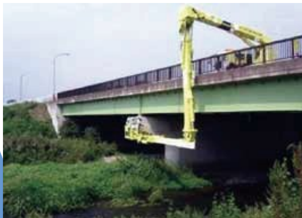
Bridge inspection example
