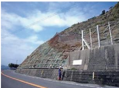
Concrete crib work
