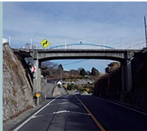
(2) Locally owned overpasses (have not been reinforced)
