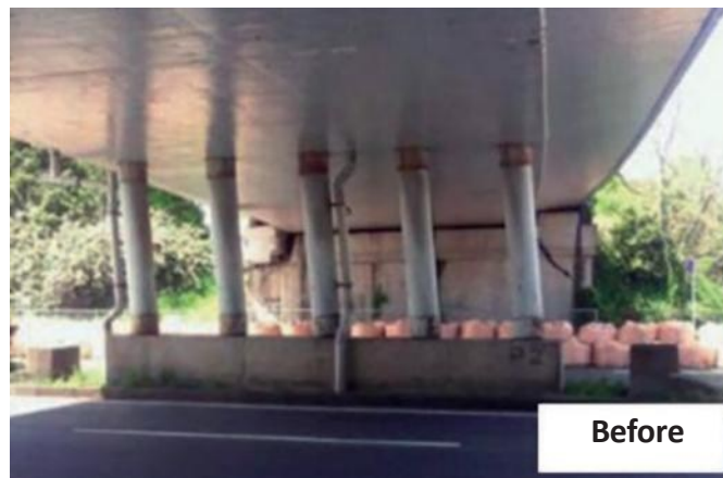
Example of seismic reinforcement
