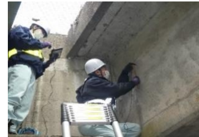
PC grout filling assessment using AE sensors
