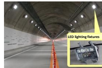
Conversion of Road Lighting to LED
