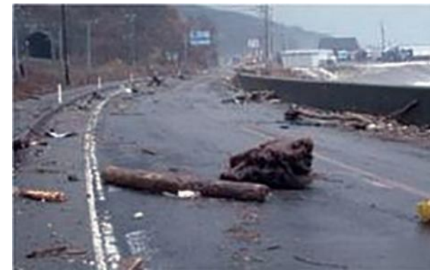
(1) Wracks from overtopping waves (On April 4, 2012 in Wasada, Tsuruoka)
