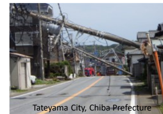
Power pole collapses caused by typhoons and other events
