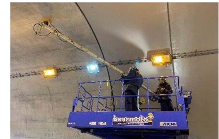
Tunnel lining deformation assessment using radar
