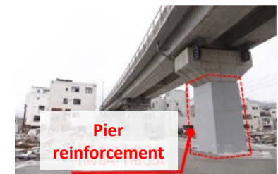
Case Study: Seismic Retrofit of the Kamaishi Viaduct
