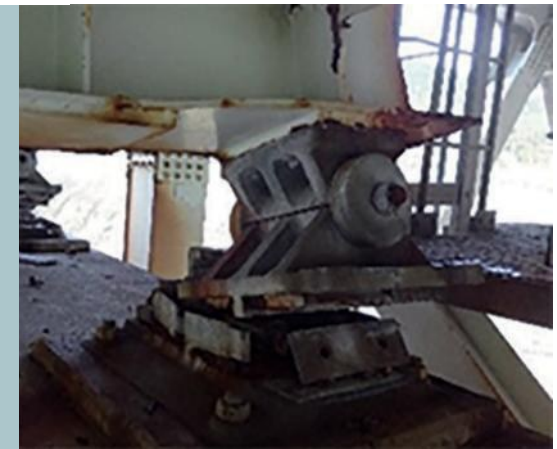
(3) Damages on supports and main girders of a bridge (Heiryu Bridge, Oita Expressway)
