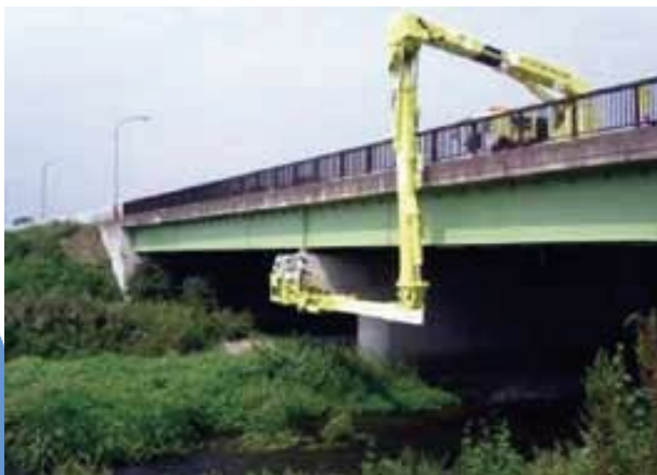
Bridge inspection example
