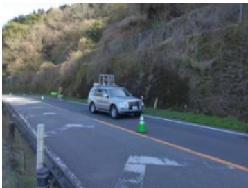
Slope and retaining wall inspection using MMS*1
