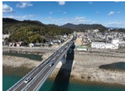
Shinmiya-Kihō Road [Opening in Fiscal Year 2024]
