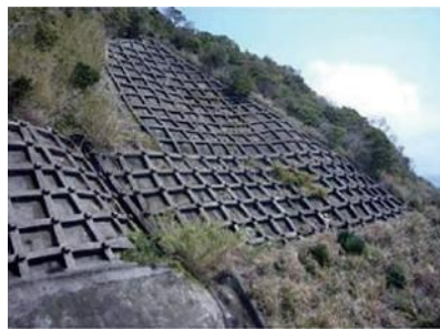
Crib work + anchoring
