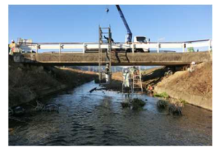
Fig.2 Demonstration of simple mobile scaffolding
