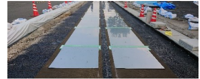
Fig. 2 Construction of transmission electrodes
