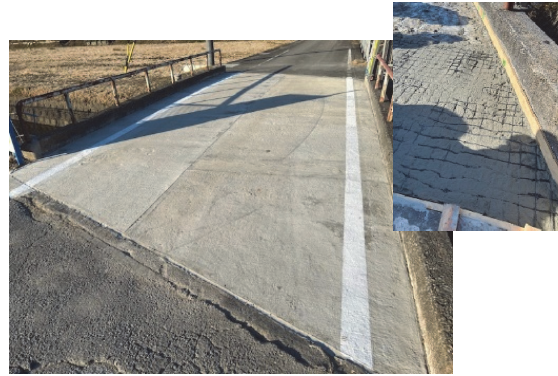
Fig. 5 On site application for bridge overlay
