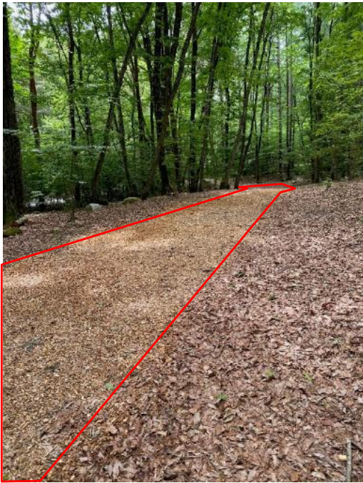
Wood Chips Made from Felled Trees Utilized for Pathway Paving (National Government Park: Alps Azumino National Government Park)
