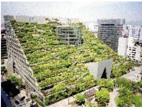
Roof Greening Project (ACROS Fukuoka)
