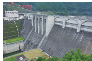
▲Concrete gravity dam (Otaki Dam)
