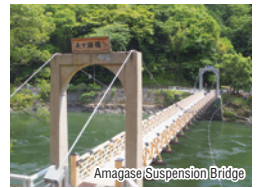
Amagase Suspension Bridge
